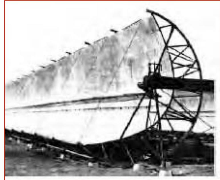
The first solar facility to produce electricity was installed in 1912 by Shuman in Maady, Egypt. The parabolic mirror trough concentrates sunrays on a line focus in which a tube was situated containing water that was brought to evaporation. It produced 55 kWatt of electric power.
